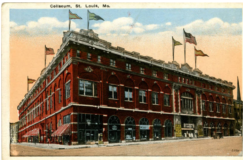
Figure 6: The St. Louis Coliseum at Washington and Jefferson Avenues occupied an entire city block, replacing the old St. Louis Exposition and Music Hall (torn down in 1907) as the city's main convention and event center (postcard courtesy of the James R. Powell Route 66 Collection, Curt Teich Postcard Archives, Newberry Library, Chicago IL).
